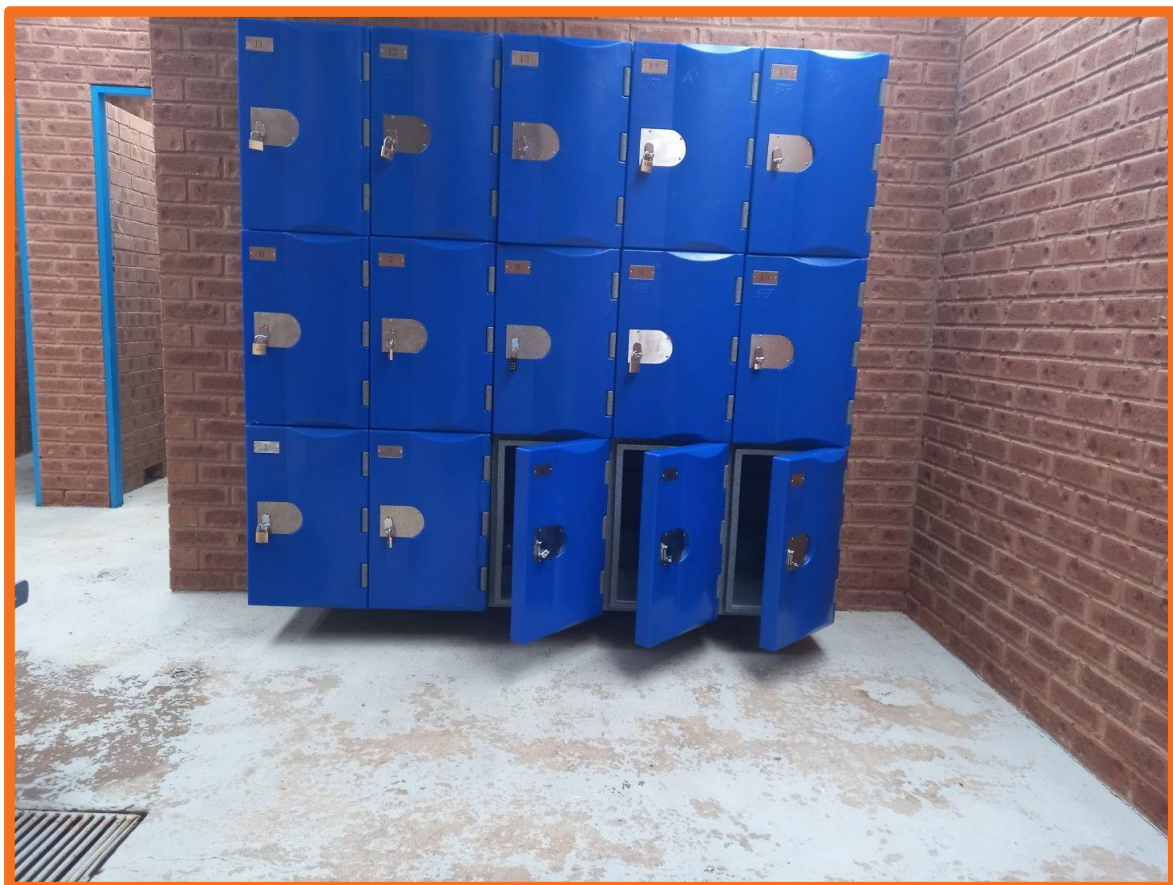
New lockers installed at the warren War Memorial Swimming Pool
